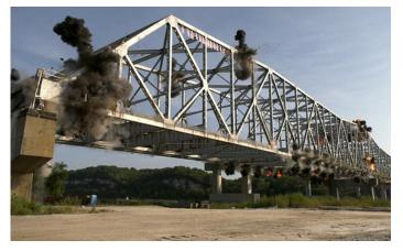
Controlled blasts demolish the old I-70 Missouri River bridge at Rocheport.
